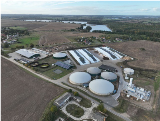
Image: Drone image of the Bio-LNG plant in Parmen
